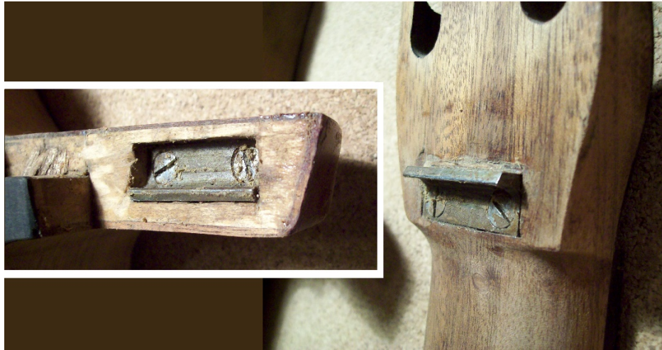
Above: The curious inner workings of the head-to-harp frame attachment that allowed for adjustment.
